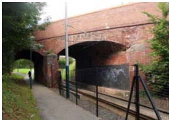
Cinderhill Rd Bridge over former colliery line
