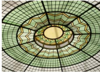
Aspley Library roof lantern
