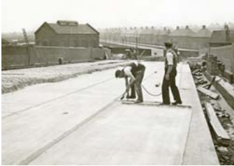
Ring road under construction during 1933*
